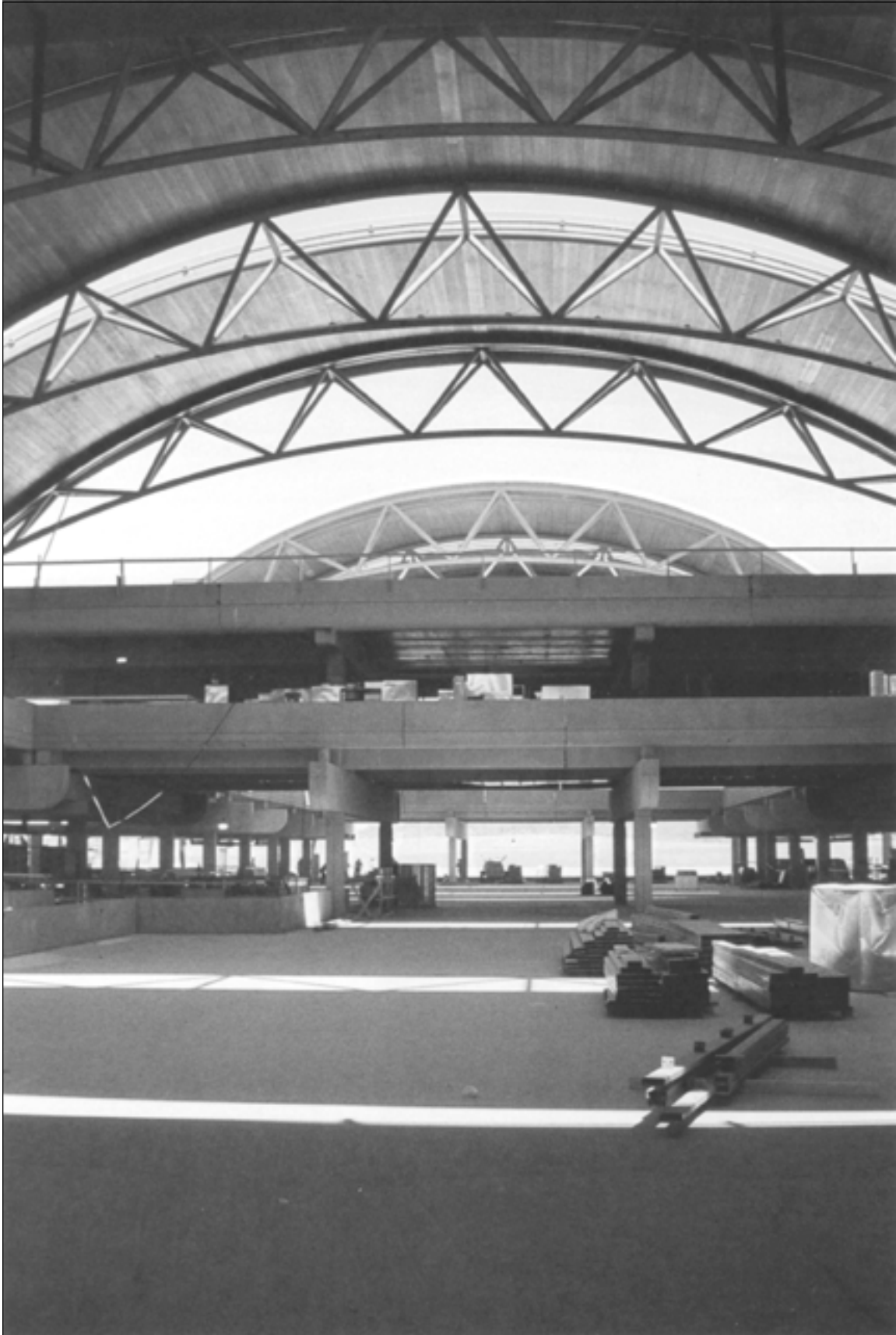
Landside Terminal of midfield complex under construction
